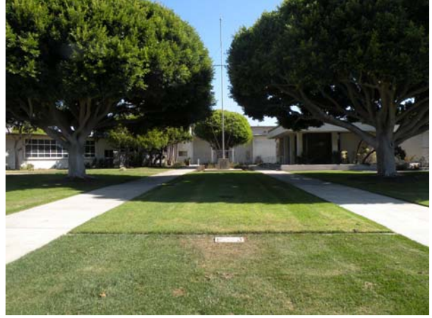
2. View of the subject property's western elevation facing east.
